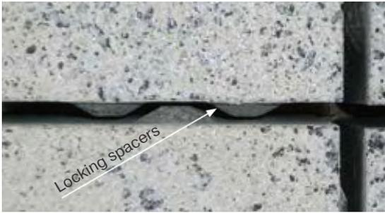
SCADA is coming with an efficient locking spacer system. This technology enables pavement to remain stable even when it is subject to strong dynamic loads, such as those generated by sudden braking of vehicles going downhill. The locking spacers are coming by size of 40 mm (VZ4) and 50 mm (VZ5), fitted on the sides of the slabs and are invisible once placed. It is not possible to combine VZ4 and VZ5.
